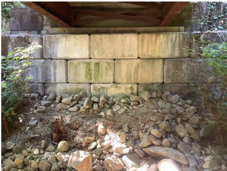
Right Bank Abutment when facing downstream
