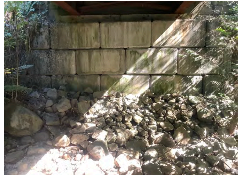
Left Bank Abutment when facing downstream
